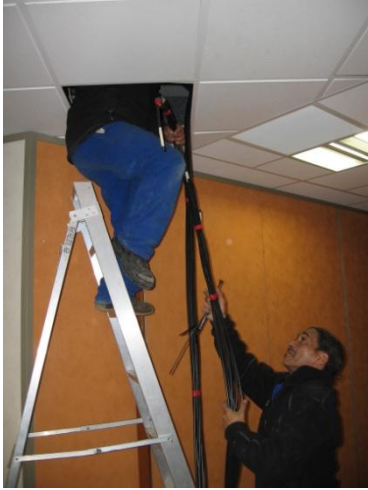
Coax cable installation. One of the sealers was attached by a seal.
